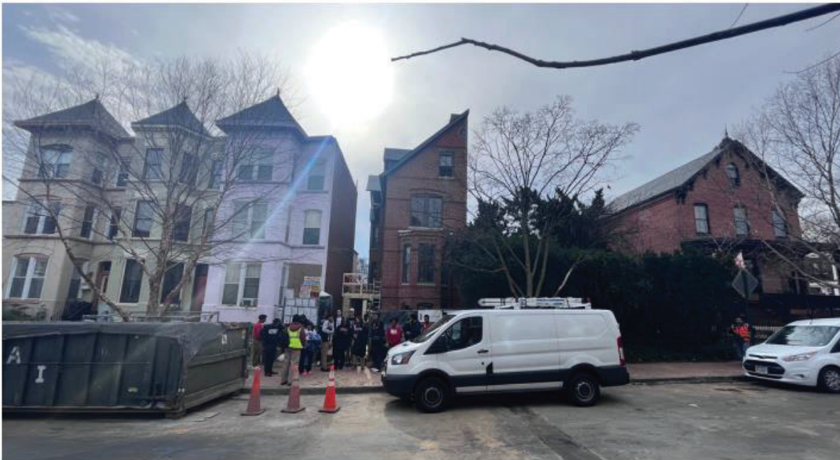
Fig. 1. The unique form of the Terrell House is the result of a devastating fire in the 1970s that destroyed its western half. (Credit: Howard University Retro Booming Team)
