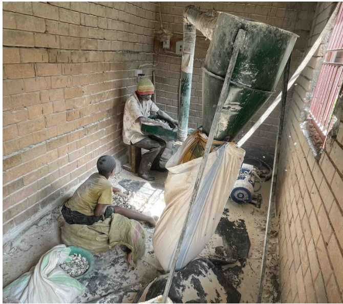
Fig. 14. The Mbaata solar mini-grid powers this milling machine used for cassava flour. The author [Which author?] left all his surgical masks behind so the operators will not breathe in fine cassava particulates. (Credit: Robert Foster)
