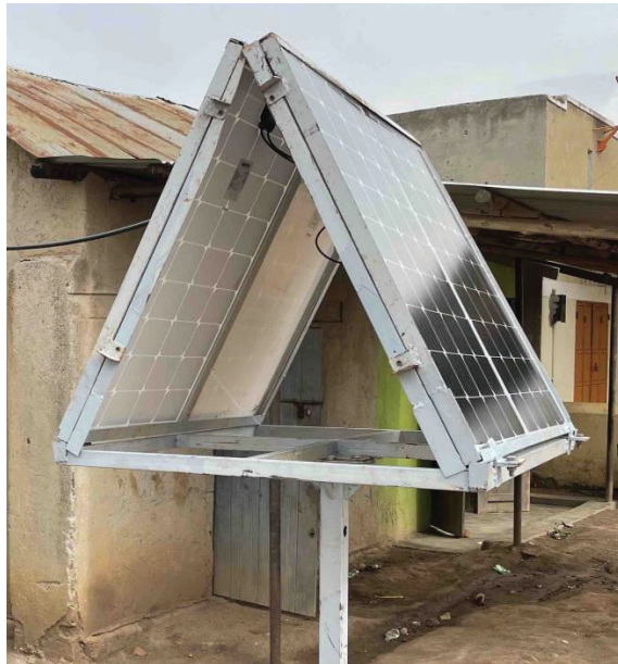
Fig. 7. A PVR Fixed E-W tracking array was installed in Katairwe village for a local convenience store that sells milk, meat, and cold drinks. (Credit: Robert Foster)
