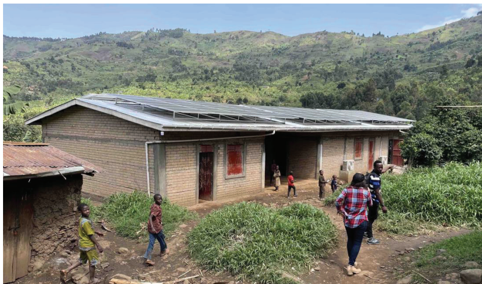
Fig. 12. The Mbaata 25-kWp rooftop solar mini-grid powers a cold room, a milling machine, a hair salon, a metalworking workshop, and a small movie theater. (Credit: Robert Foster)
