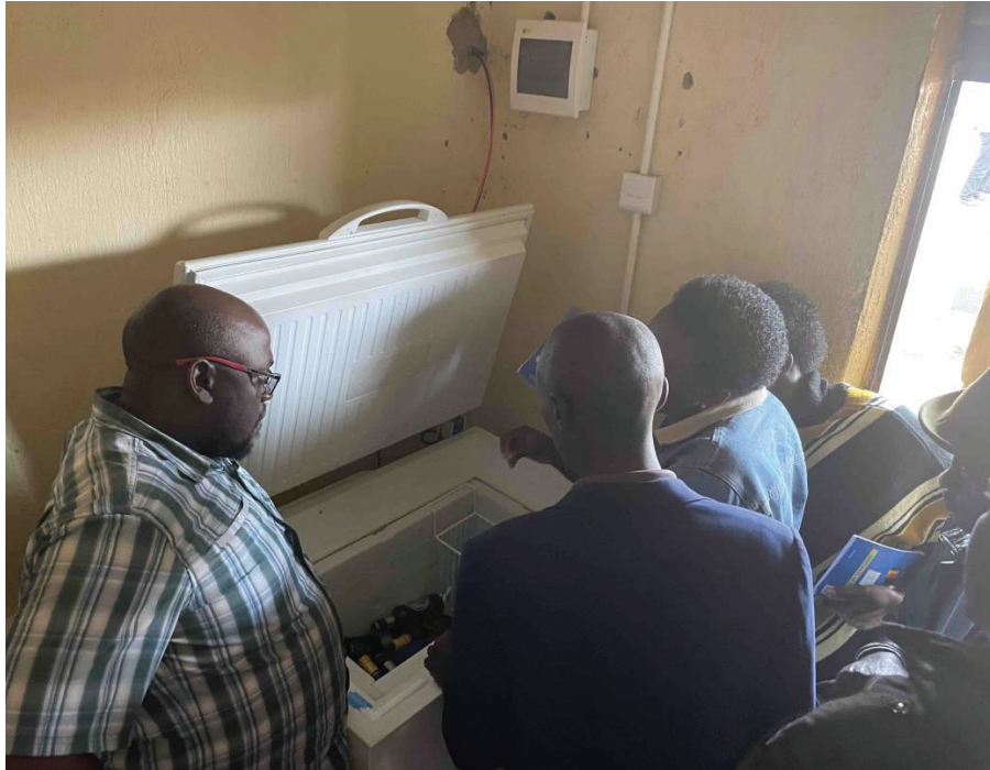
Fig. 11. Local Katairwe farmers during a USDA-sponsored PURE training event inspected a direct-drive PV refrigerator (PVR) with thermal storage used by a store to preserve meat and chill milk and drinks. (Credit: Robert Foster)
