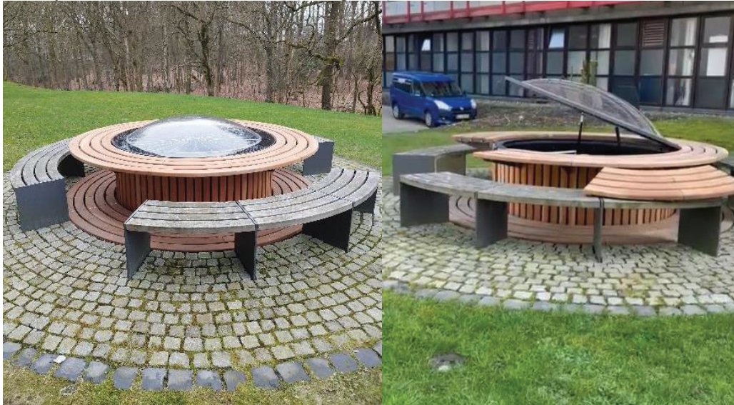
Figure 5: GeoStar 2 entrance to the distribution shaft
