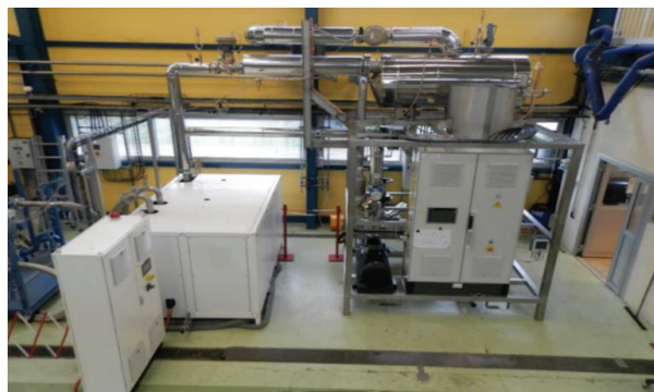
Figure 1: Test Bench in EDF Laboratory
