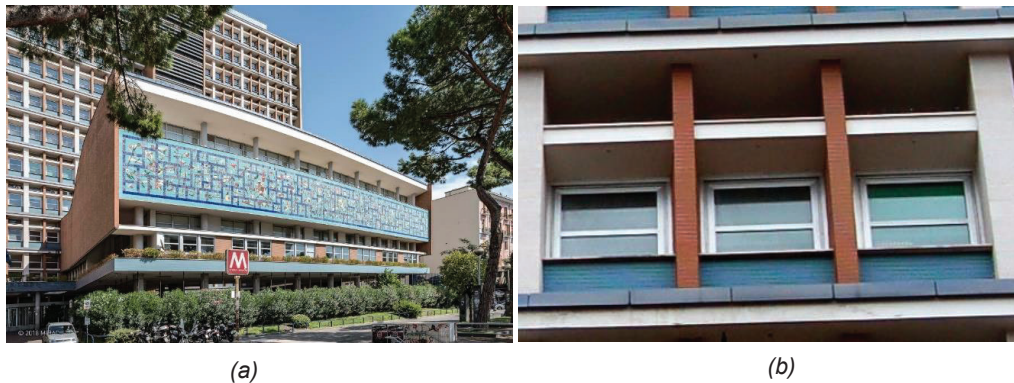
Figure 2. University of Federico II, Piazzale Tecchio, Naples, Italy (a), Investigated Office (b)
