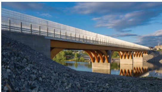
Figure 16: Mistissini Bridge (Courtesy of Stantec)
