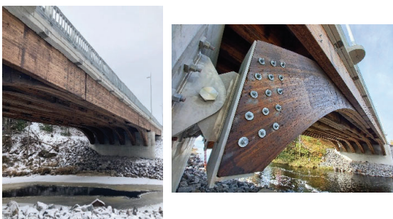
Figure 17: Duchesnay Creek Bridge (Courtesy of MTO)
