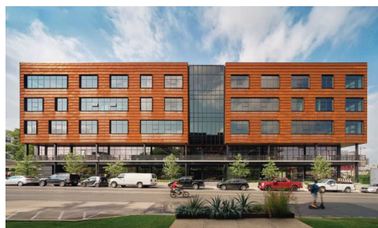
Figure 3: 901 East Sixth, Austin, Texas; Architect: Thoughtbarn and Delineate Studio; Engineer: Leap Structures
