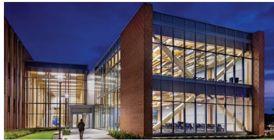
Figure 10: Anderson-Ball Classroom Building, San Jacinto College, Pasadena, Texas; Architect: Kirksey; Engineer: Armstrong-Douglass Partners
