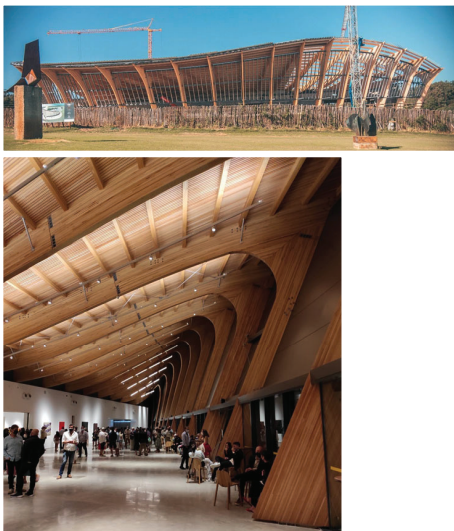
Figure 13: Images during the construction process of MACA
