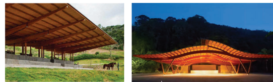
Figure 4: Eucalyptus glulam structures in Brazil [12]
