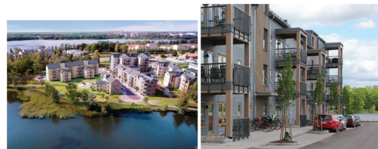
Figure 7: Arken (CLT 4) constructed in CLT in Växjö, Sweden
