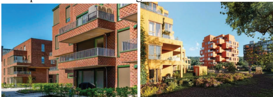
Figure 4: Ski BB1 Magasinparken project (Concrete 1) built with concrete in Ski, Norway
