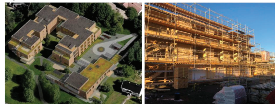
Figure 2: Solhøy project (CLT 2) constructed with CLT in Vestby, Norway
