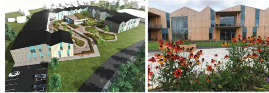
Figure 1: Bergheim bo- og aktivitetssenter project (CLT 1) constructed with CLT in Halden, Norway
