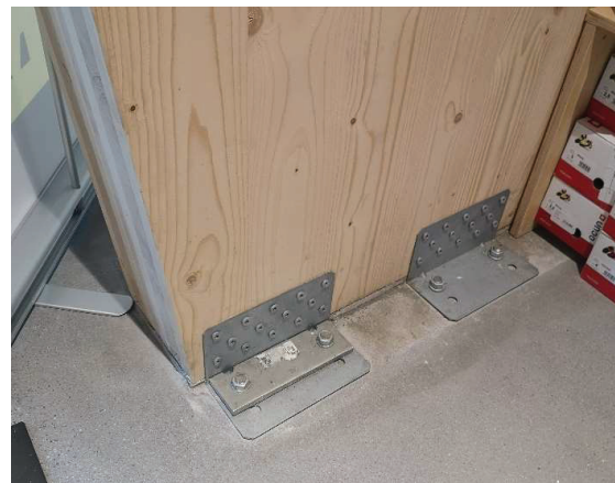
Figure 13: Proprietary angle bracket to base of portal frame
