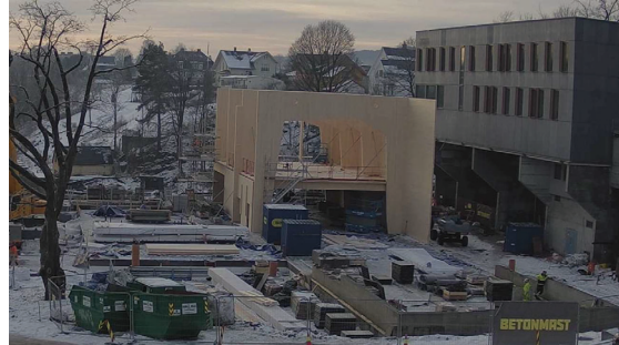
Figure 22: HUT under construction – climbing hall
