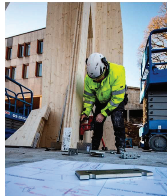
Figure 24: Installation of steel brackets between timber and concrete
