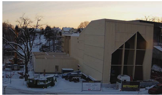
Figure 23: HUT under construction – annex building
