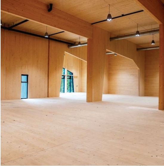
Figure 25: Finished building before fitting out
