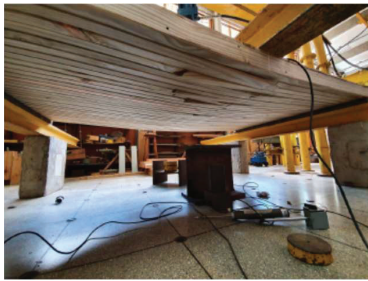
Figure 8: NLT panel rupture details
