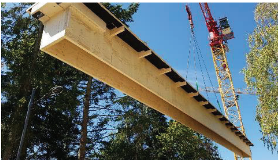
Figure 16: A prefabricated 23,75m roof element on the crane
