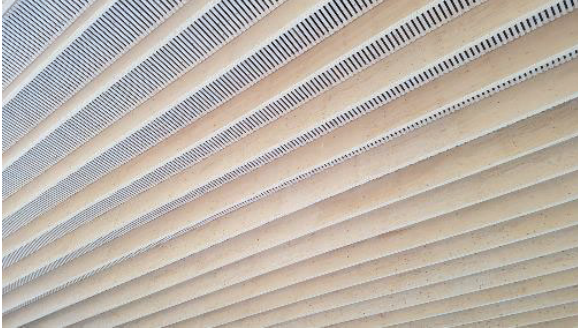
Figure 20: Roof underside with acoustic ceiling and LVL-Panels in visual quality
