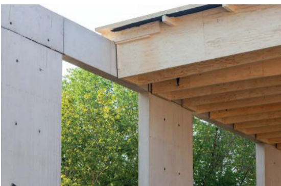
Figure 11: Finished notched support of the PI-beams on the concrete ring.
