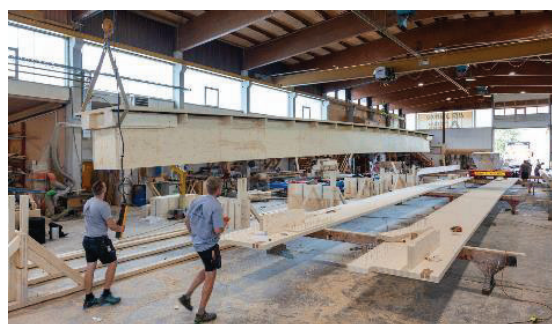
Figure 13: Production of the PI-elements in the factory
