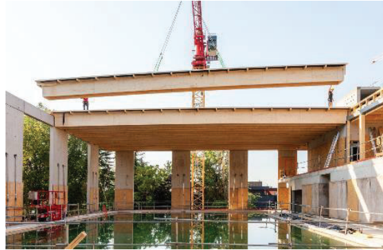
Figure 17: Assembly of the roof with individual LVL PI-Panels
