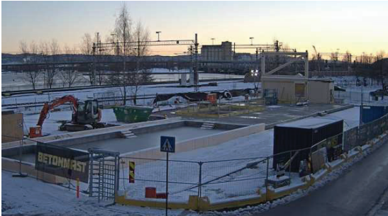
Figure 26: Start of timber erection
