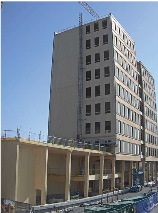
Figure 27: Completion of timber erection
