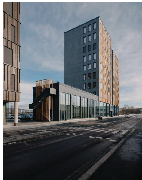
Figure 29: SporX – finished building
