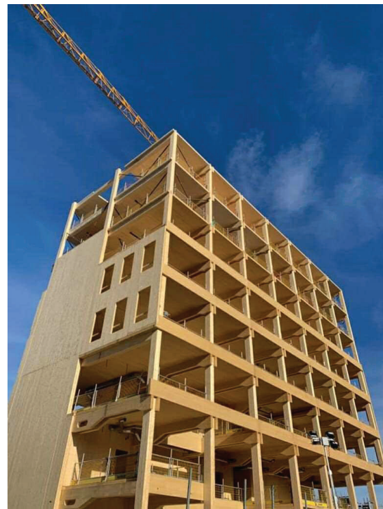
Figure 5: SporX under construction showing the exposed structural frame
