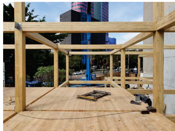
Figure 18: First wood building in Brazil – under construction.
