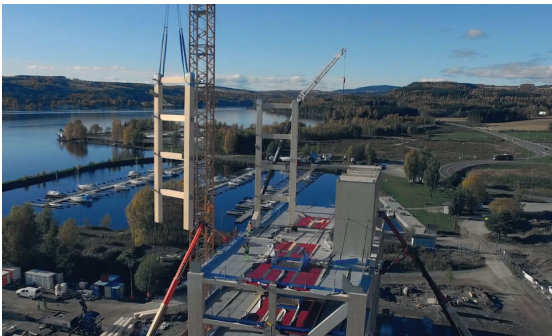
Figure 16: Hoisting of frames.
