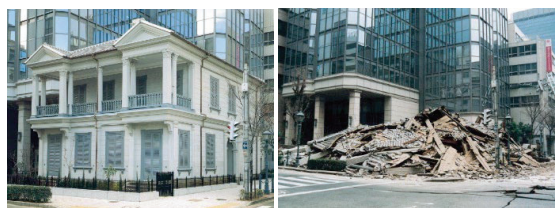
Figure 4: The Jugobankan Building before (left) and after (right) the Kobe Earthquake (1995) [4]
