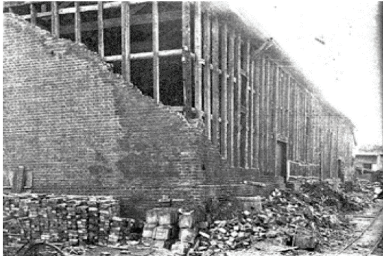
Figure 3: Damage to TFBC building during Tokyo-Yokohama Earthquake (1923) [3]
