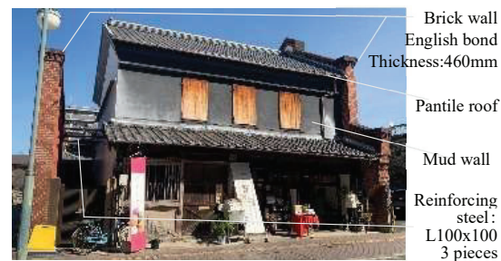
(a) South (front) exterior
