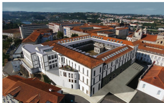
Figure 2: 3D view of the designed building at the end of the works
