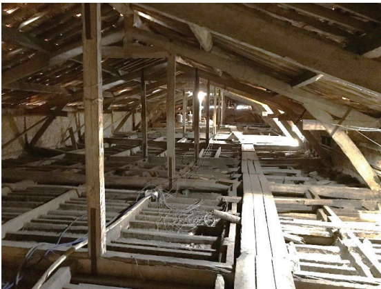
Figure 7: Floor structure under the roof
