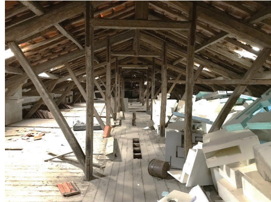
Figure 4: General view of the roof
