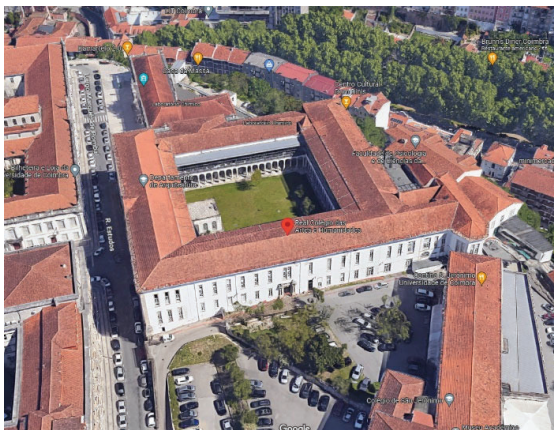
Figure 1: General view of the building
