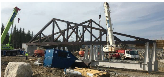
Figure 13: Trusses after erection. Photo: Viggo Jakobsen, Consto Nord AS
