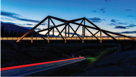
Figure 3: Skytebanen bridge by night. Photo: Jan Inge Larsen
