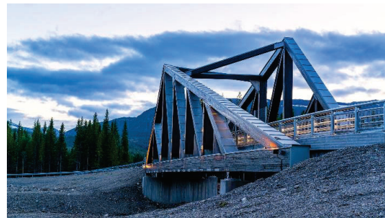
Figure 2: The bridge seen from the east side. Photo: Jan Inge Larsen
