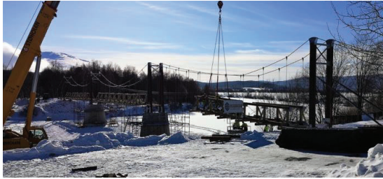
Figure 12: Bridge erection (lateral span)
