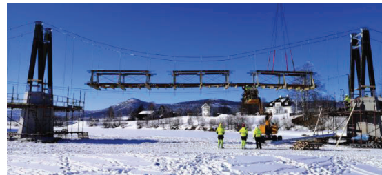
Figure 11: Bridge erection (central span)
