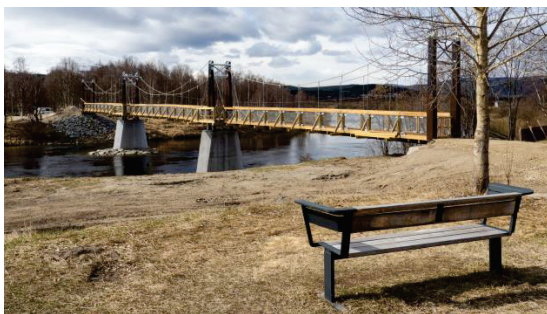
Figure 1: View of the Neby pedestrian bridge
