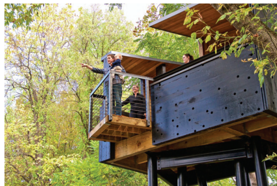
Figure 1: View from railroad of completed tower
