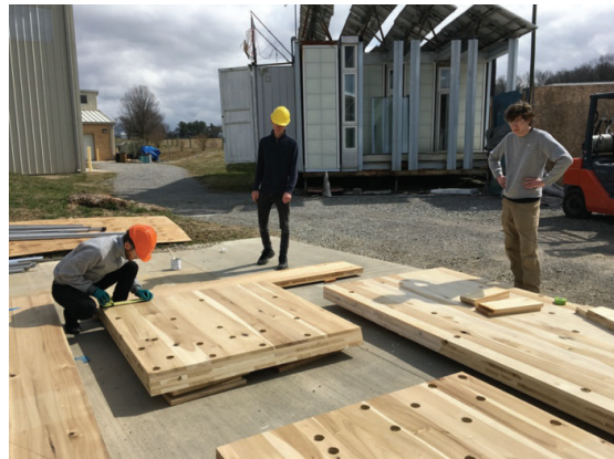
Figure 7: Yellow Poplar CLT panels before surface treatment
