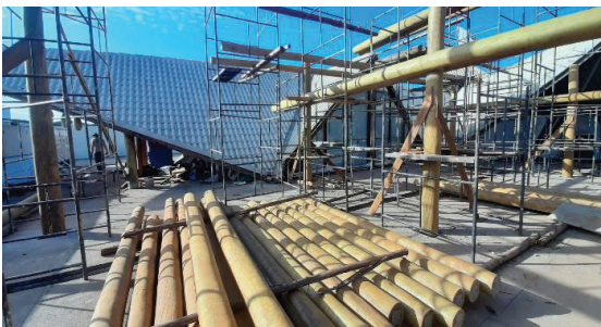
Figure 4: Assembling of the timber structure over the existing concrete slab
