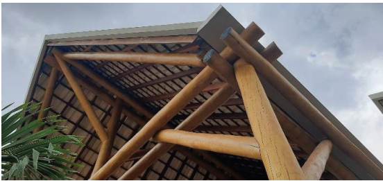
Figure 11: External view of the finished wooden pole structure
