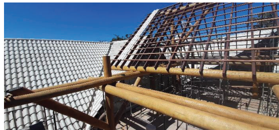
Figure 7: Execution of the covering
