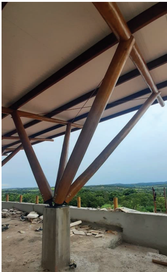
Figure 25: Internal view of the pole frame
