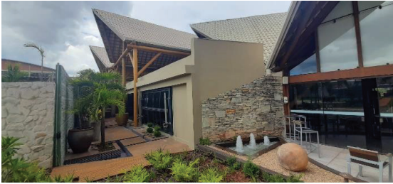
Figure 10: External view of the buildings
