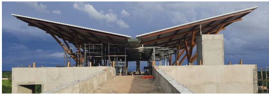
Figure 23: External view of the spatial structure of the winery
