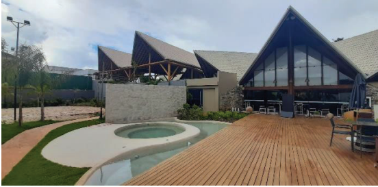
Figure 9: External view of the buildings
