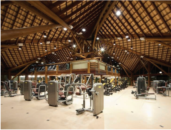
Figure 2: Internal view of the wooden building
