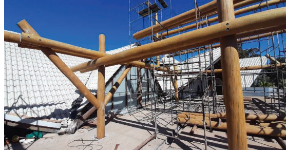
Figure 5: Assembling of the timber structure
