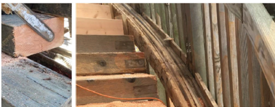
Figure 8. replacement of end parts of the stairs
