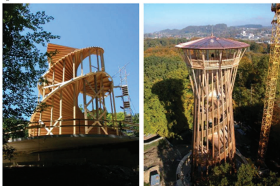
Figure 7. Construction of the tower, 2003
