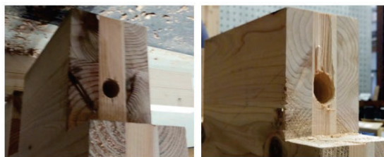
Figure 10: Through hole in CLT before and after modification
