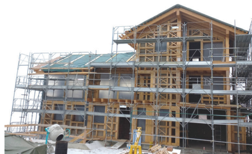
Figure 4: On construction site: Nidus modules assembled
