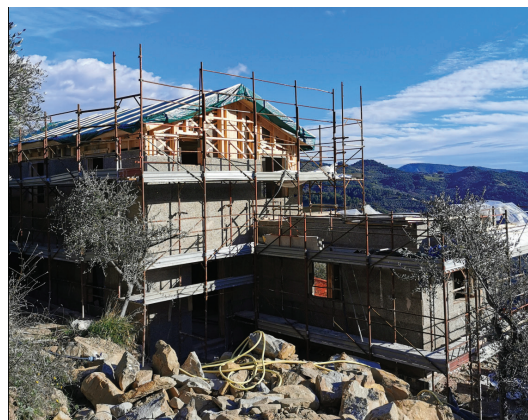
Figure 1: Example of timber-mortar constructive system use; prefabricated only-timber frames assembled on-site (above) and building during the pouring of lime mortar (below)
