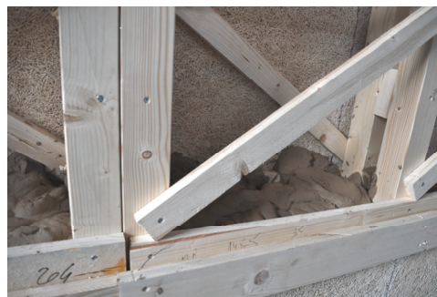
Figure 5: Detail of Nidus wall during mortar casting
