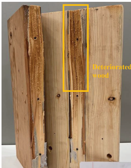
(b) Failure plane of SG-04
