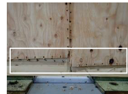
Fig 3.13: Nail punching out hand-tightened and 20 kN
