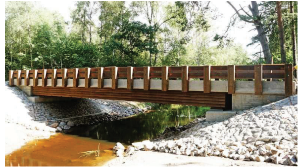
Figure 11: Jecupe bridge in a construction stage and in a finished state
