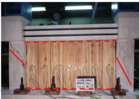
Figure 2: Column shear failure as observed in [3]
