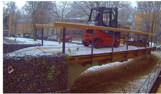
Figure 12: Load application for a long-term test with a fork lift
