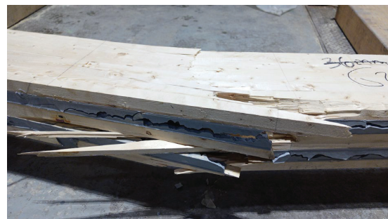
Figure 6: Damaged reinforced beam
