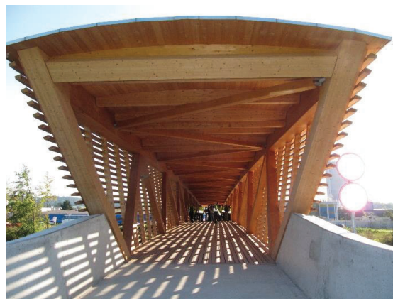
Figure 7: Swiss timber bridge structurally protected by a roof and an open cladding (photo: A. Simon)
