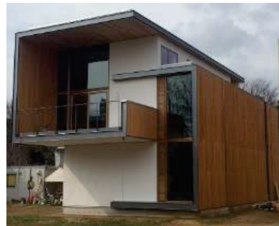
Photo 4. 2-story CLT test house in BRI.
