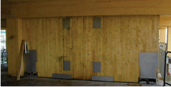
Figure 5: Shear wall with hold-down connected to the concrete mezzanine
