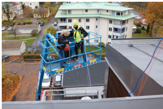
Figure 7. Installation of cables and accelerometers in progress using a 25 m sky-lift.
