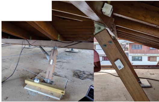
Figure 5: Monitoring 3 wood elements (softwood and hardwood) equipped with sensors in Cayenne.
