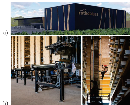
Figure 1: View of Rotho Blaas ASSTW: a) external view, b) internal view with automatic lifting system.
