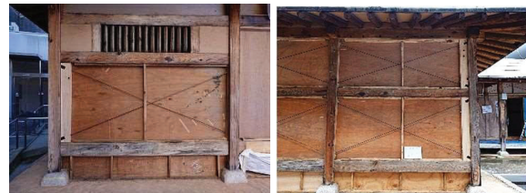
Photo 3: Appearance of the target building (After reinforcement)
