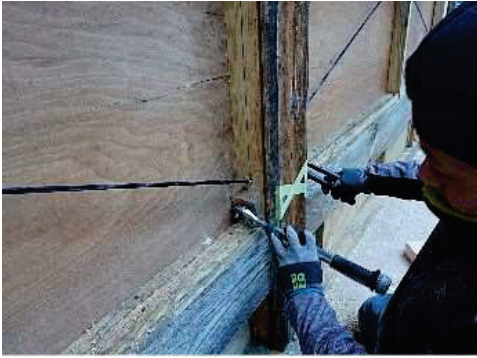
Photo 5: Control of tightening torque
