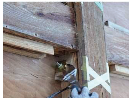
Photo 4: Control of tightening torque
