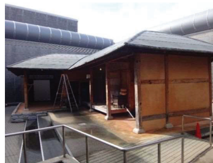
Photo 1: Appearance of the target building (Before reinforcement)
