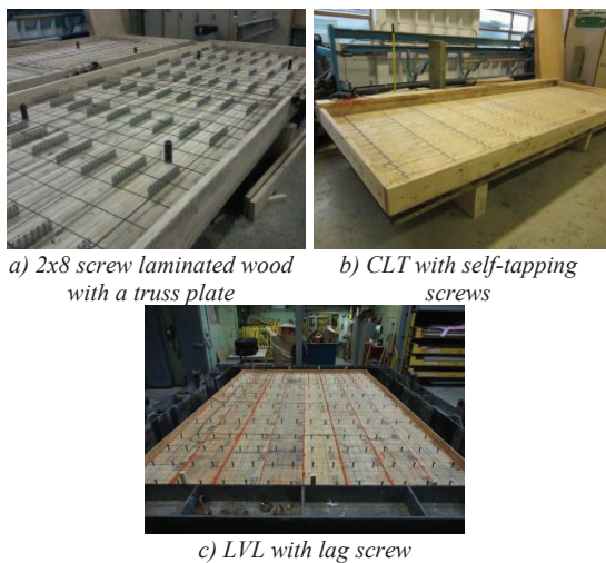
Figure 4: TCC floors under construction for fire-resistance testing
