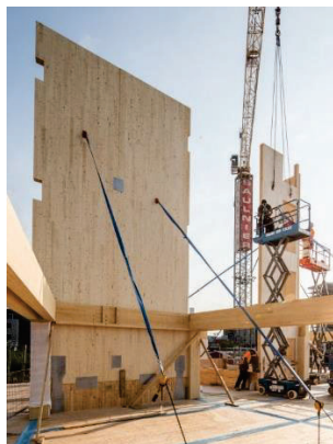
Figure 1: Example of a balloon wall in CLT construction
