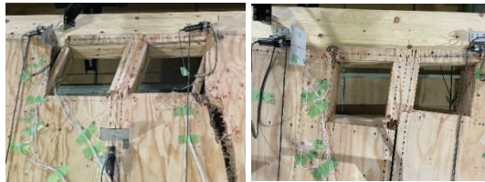
Figure 16: Failure of upper opening
