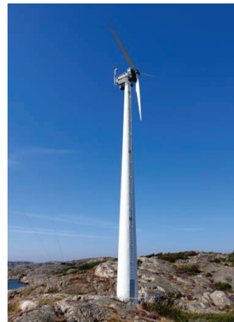
Figure 1: Demonstrator of the wooden wind turbine tower used for research on Björkö island near Gothenburg, Sweden
