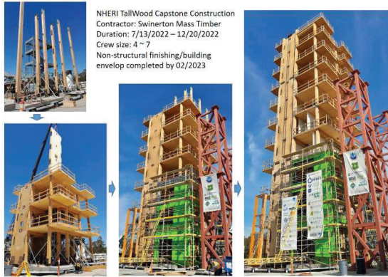
Figure 5: Construction process of the test building
