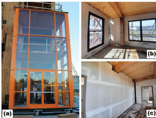
Figure 6: Selected non-structural systems and components included in the test (a) Curtain wall (b) Exterior wall and windows (c) Interior partition walls.
