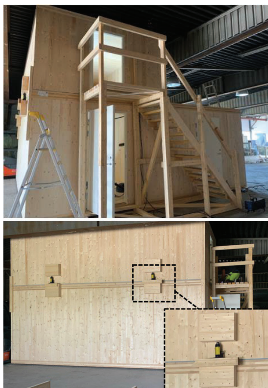
Figure 1: Test room set-up.
