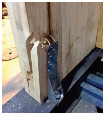
Figure 14: Damage in HD_1 connector after 100kN lateral load.
