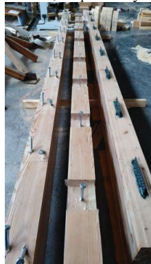
Figure 3: Installed connectors on the timber beams
