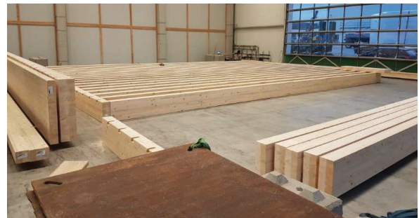
Figure 5: Beams are positioned.
