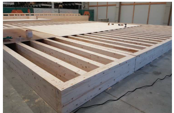
Figure 6: Three-layer boards are glued on.
