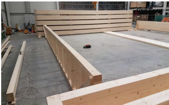
Figure 8: The supporting wall is built.
