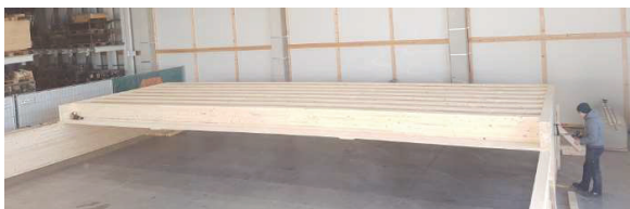
Figure 9: Elements are turned and laid on the wall.
