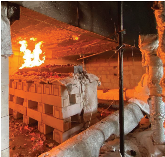
Figure 14: Bond-line failure leading to premature char fall-off in experiment with beam. Detached char is apparent on floor and burner.
