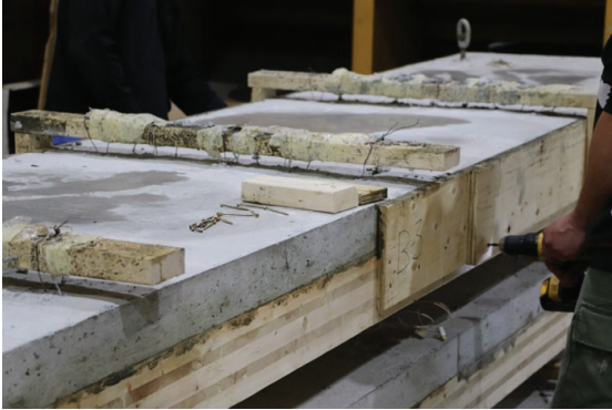
Figure 5: Removing formwork from TCC floor slabs
