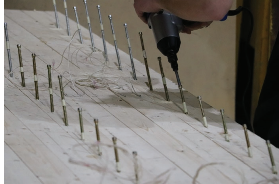
Figure 2: Installation of STS in CLT Panel
