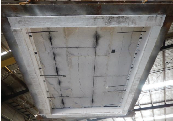
Figure 2: Exposed face of specimen at the end of the monitoring period.
