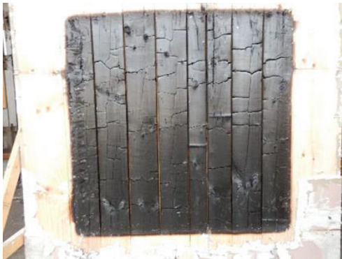
Figure 10: Underside of CLT panel with plasterboard removed after 23-hour monitoring period.
