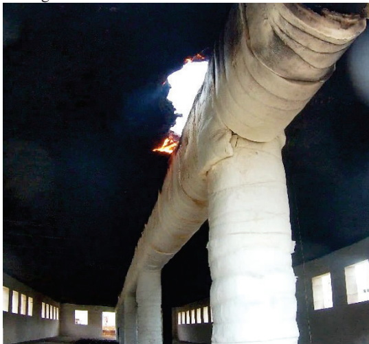
Figure 7: CLT ceiling smouldering hotspot 40 hours after flames, forming a hole in the CLT. Transition to flaming is also observed.
